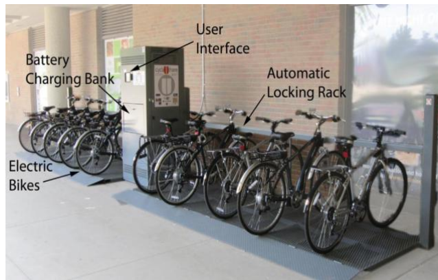
Figure 3: Components of e-bike sharing system station [8]
